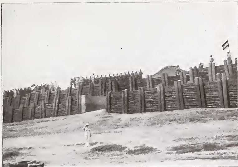
55. Pile defences of the station at Kusseri against the floods of the Logone.
